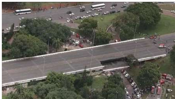
Figure 4 - Upper view of the viaduct instants after partial collapse, source: public
