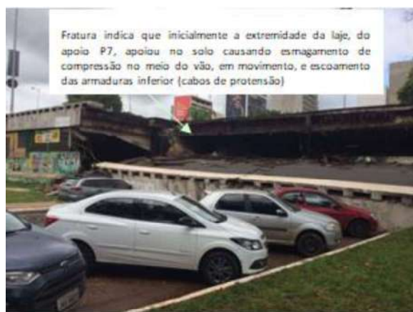
Figure 3 - Situation of the spaces underneath the viaduct, Source: public
