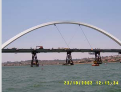
Phase a – 4 hangers in the central arch
