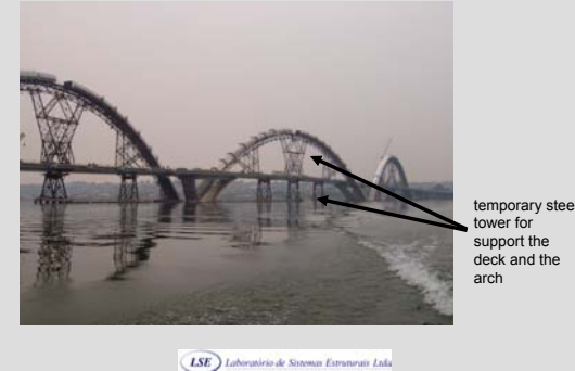
Metallic structures over the deck for the construction of the arches
