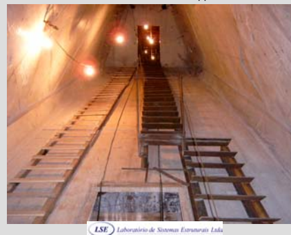
hollow box made of concrete for support the steel arch
